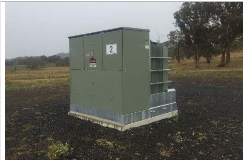
Plate 2.4 – Kiosk type transformer near base of tower for Turbine 2.
